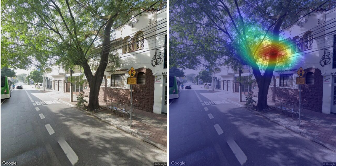
Figure 1: (Left) Image of a tree with branches and leaves in contact with overhead powerlines. (Right) The corresponding Grad-CAM++ image, showing (in red) that the whole extension of the wires passing through the tree canopy has been identified and relevant for classifying this image (as a true positive) by the DLN used.
